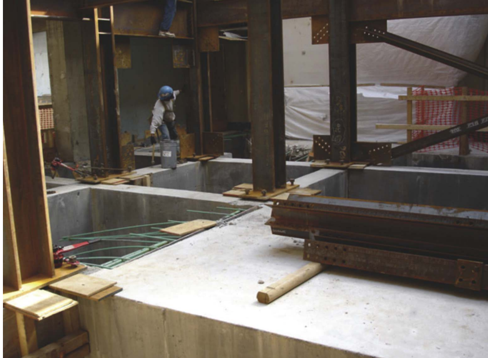
The new elevator bank's pit walls function as girders carrying new structural steel columns and lateral bracing.
