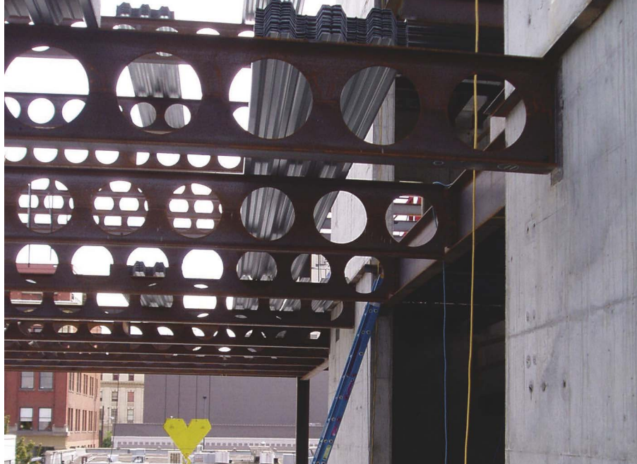
Cellular beam web penetrations were aligned from beam to adjacent beam, allowing services to be easily run in the ceiling cavity.
