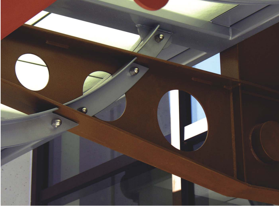
The cellular-beam appearance is mimicked in structural steel details for the exterior entrance canopy.
